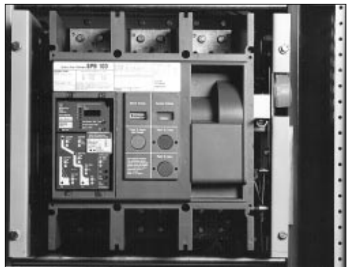
Figure 3-2 Insulated Case Circuit Breaker
