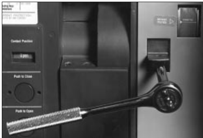
Figure 6-1 Drawout with Socket Wrench
