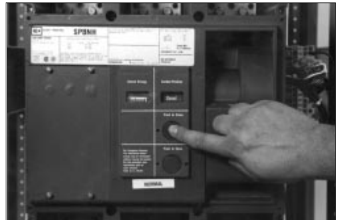
Figure 5-2 Close Switch by Pushing Close Button
